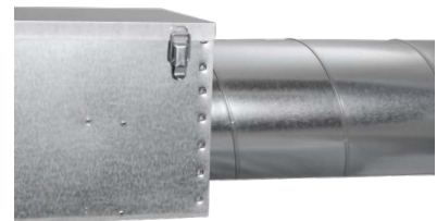
3. Install the filter box on the opposite duct hole.
