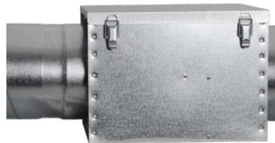
4. Insert the SMSFL coupling. Use WGO self-drilling screws to secure the installation.
